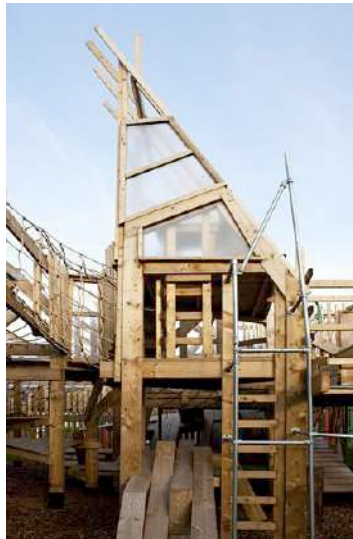
Made with standard treated timbers, key clamps and steel tubing
